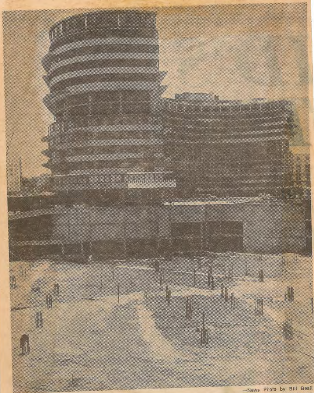
SPROUTING — These prongs are on the pilings for the foundations of the next stage of the Watergate Town project—a “T” shaped high rise combination office building and hotel. Behind them is the nearly completed 13-story Watergate East cooperative apartments, off Virginia-av and Rock Creek Parkway. The office building-hotel is scheduled to open in mid-1966.
