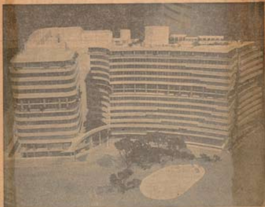
Construction work has begun on this $10 million, two-building complex in the Watergate project in Foggy Bottom. The Watergate office building (left) is joined to the residential hotel by a service core and walkways.
